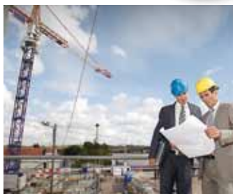
Bridging a gap Preservation and pest control in buildings from the outset
